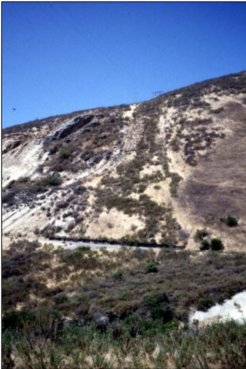
After repair, vegetation beginning.
