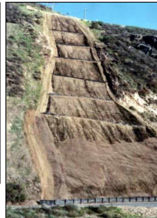
Slope immediately after infill of cells.
