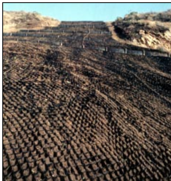
Sections of GEOWEB were stapled together for this large expanse of slope and anchored with metal stakes.
